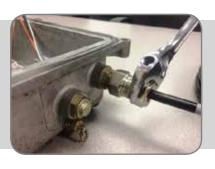
Push the rear piece of the node entry connector up the cable, and thread onto the front piece. Use a wrench to tighten, and make sure the cable is firmly in place and does not slide when pulled on. Take caution to not over tighten the connector, it could cause damage to the connector threads or the cable itself.
