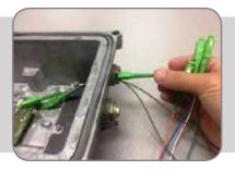
Start by placing the connectors into the node housing one at a time until all connectors are inside the node housing.
